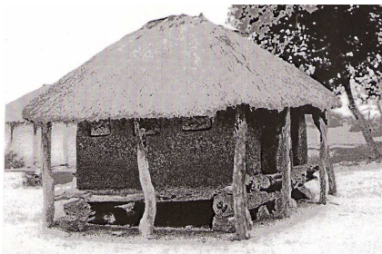
Gridiron varieties of the Granary using adobe and wood and concrete blocks
