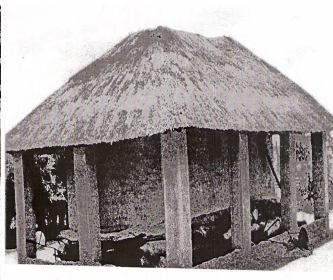
Gridiron varieties of the Granary using adobe and wood and concrete blocks
